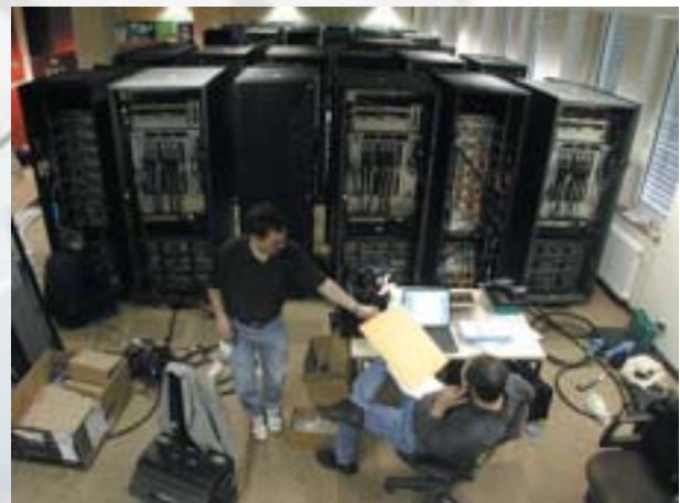
Figure 2: The installation phase of HLRN at Hannover
