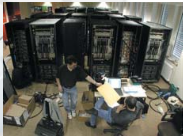
Figure 2: The installation phase of HLRN at Hannover
